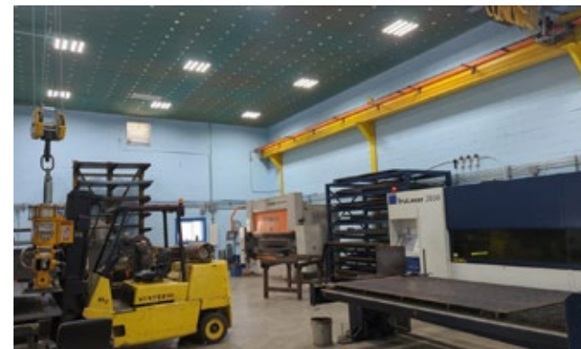
Metal Fabrication Shop Ceiling Mounted (6500K - No Lenses)
