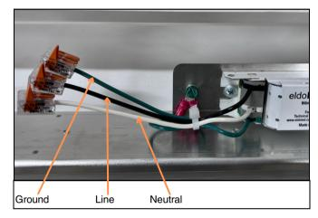
**3.** Confirm all wires are firmly connected to their respective spots. Test light to ensure functional operation.
